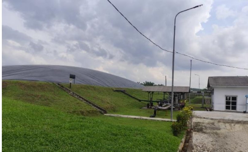
Gambar 2. Anaerobic Bio digester sistem CIGAR ( Covered In Ground Anaerobic Reactor )
