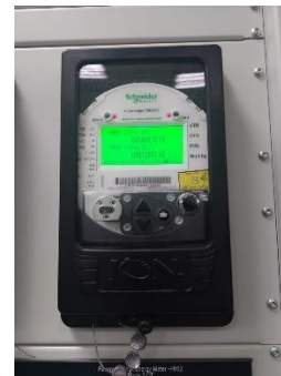
Gambar 6.3. Panel Room (kWh Meter)
