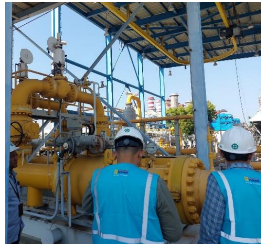
Gambar 6.7. Gas Metering & Fuel Gas System
