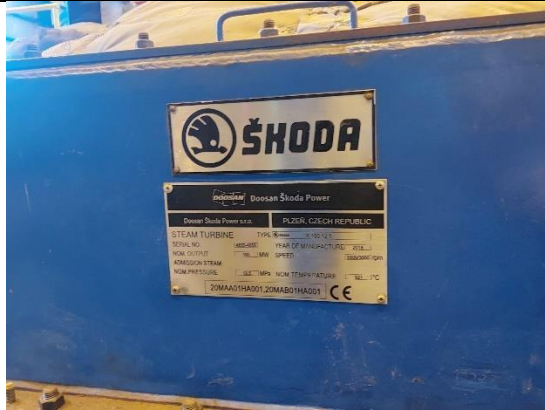
Gambar 6.4. Steam Turbine
