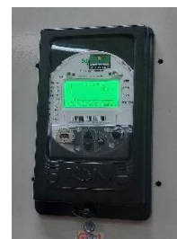
Gambar 6.3. Panel Room (kWh Meter)
